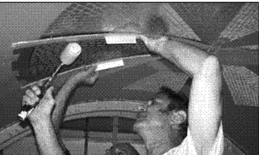
The mosaic is applied utilizing a stencil and then applying adhesive using a paint roller.
