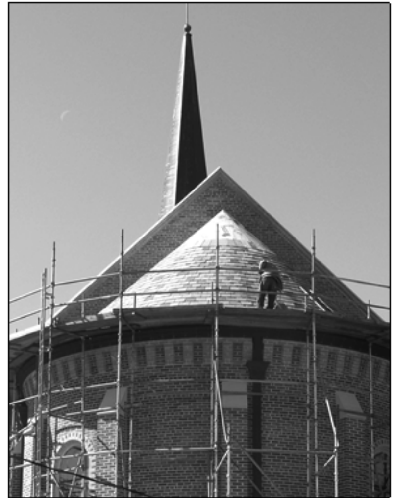
The roof area above the apse is almost complete.
